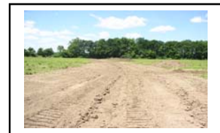
West Homes-Crosby Township. "Before" Waterway installation.
