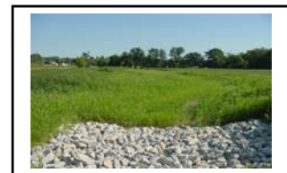
"After" Waterway installation.
