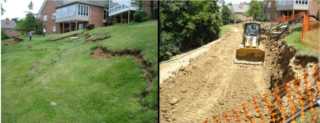
Typical residential landslide (left). Engineered repair of same (right).
