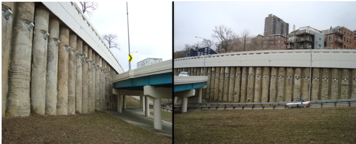
The Mt. Adams Retaining Wall.
