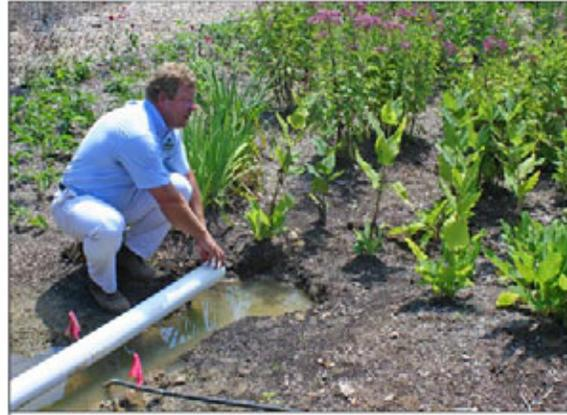
Fig. 4 Rain water piped from downspouts into a rain garden
