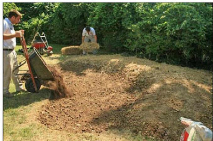
Fig 9. Adding soil and amendments to a rain garden
