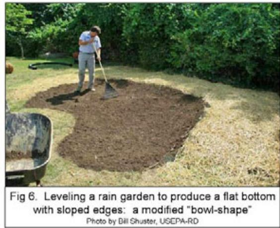
Fig 6. Leveling a rain garden to produce a flat bottom with sloped edges: a modified "bowl-shape"
