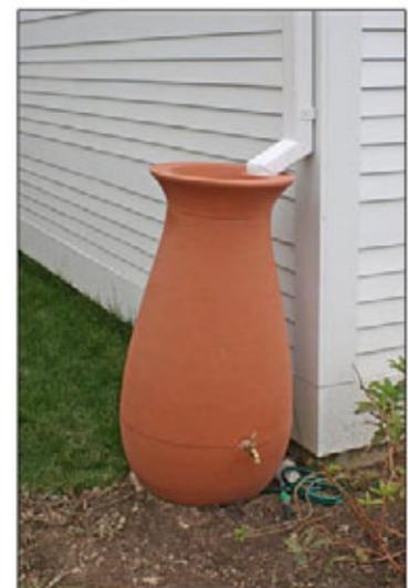
Fig. 5 Rain barrel collecting water from a downspout
