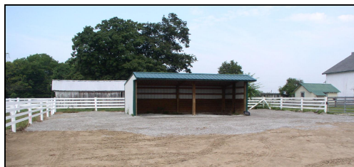
EQIP Program Heavy Use Area around a pasture shelter
