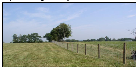
EQIP Program Woven wire fencing project completed
