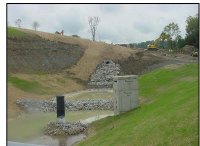
Western Ridge Development sediment basin
