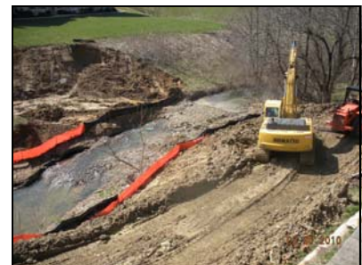
Glenbridge Manor stream relocation
