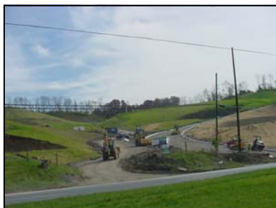
Western Ridge Development stabilized hillsides
