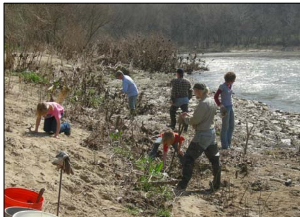
Planting of willow stakes along river bank at Colerain Township's Heritage Park
