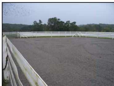
EQIP Program Completed gravel heavy use area
